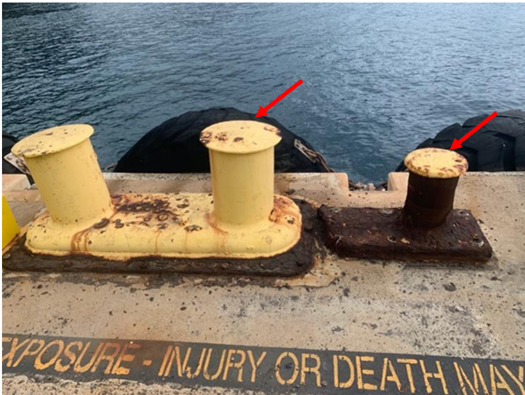
Photo 6: Two Bollards at Approx. DM 385 to be Demolished and Removed
