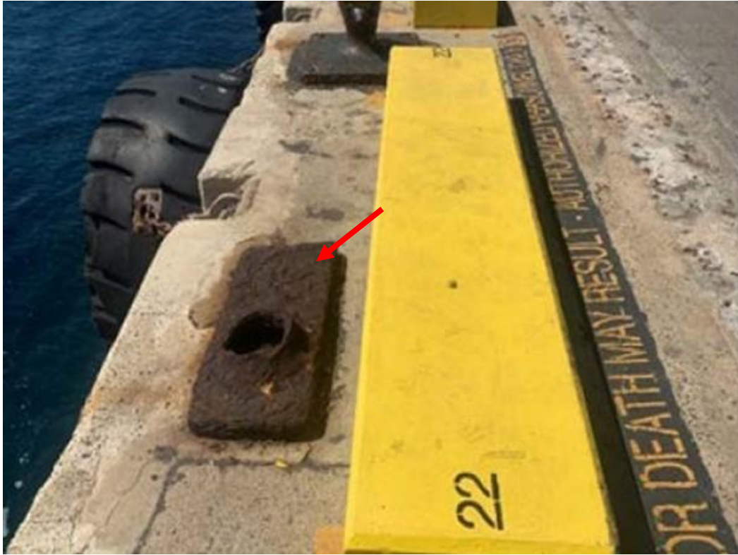
Photo 5: Bollard at Approx. DM 230 to be Demolished and Removed.
