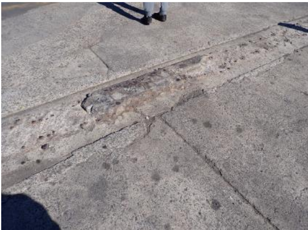
Photograph 2: Typical Rail Footing to be Demolished and Removed.
