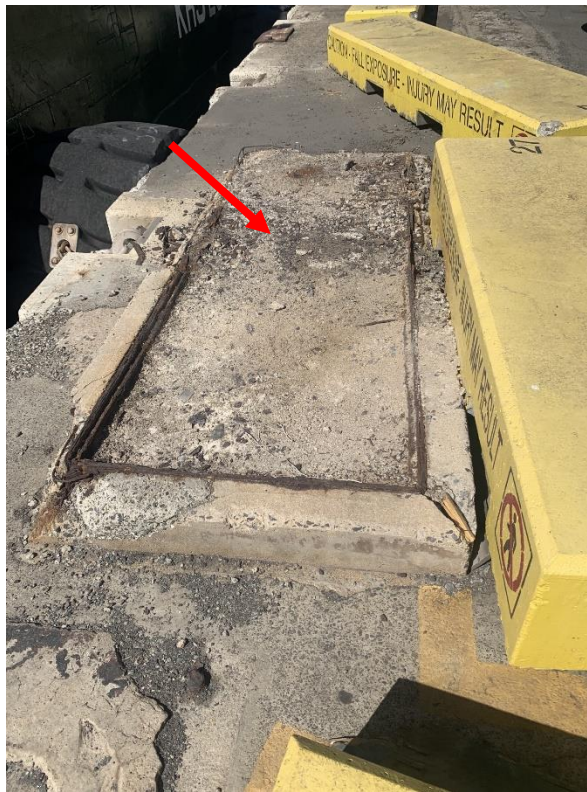
Photograph 8: Concrete Footing & Railing to be Demolished and Removed.
