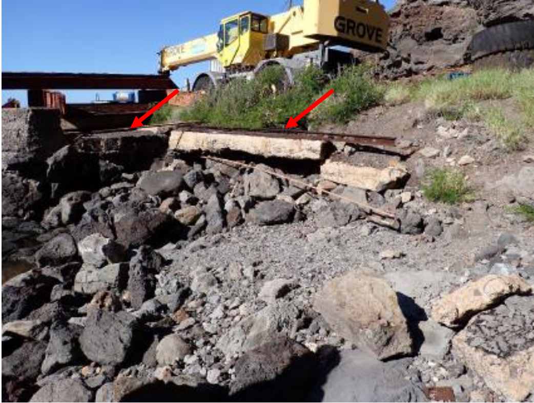
Photograph 3: Rail Footings on Grade to be Demolished and Removed
