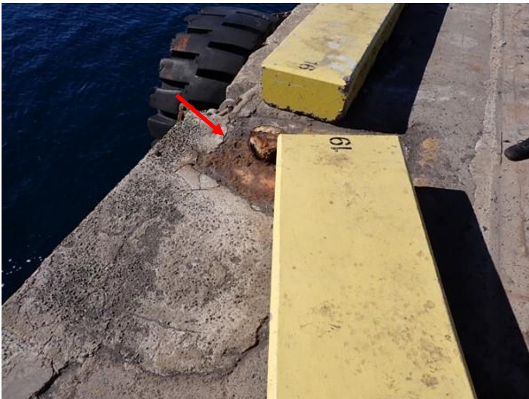
Photo 4: Bollard at Approx. DM 200 to be Demolished and Removed
